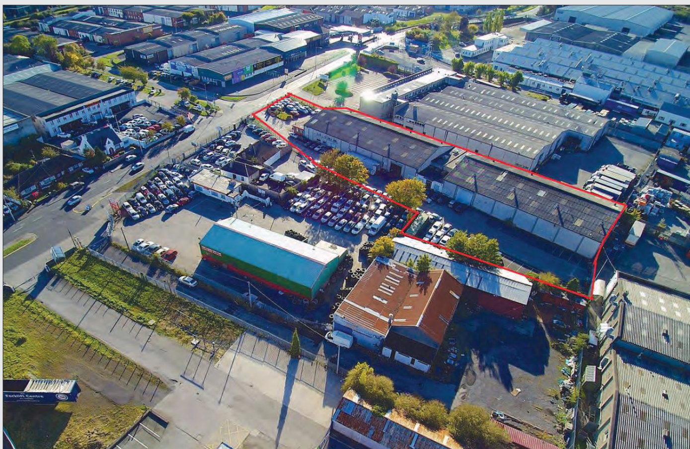
OLDER-STYLE: The industrial unit in Ballymount which is an attractive location
