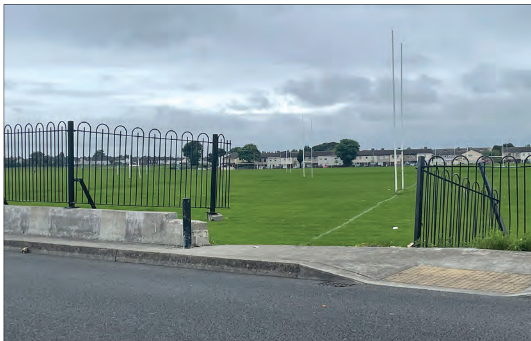
REPAIRED: The boundary fence damaged at McGee Park
