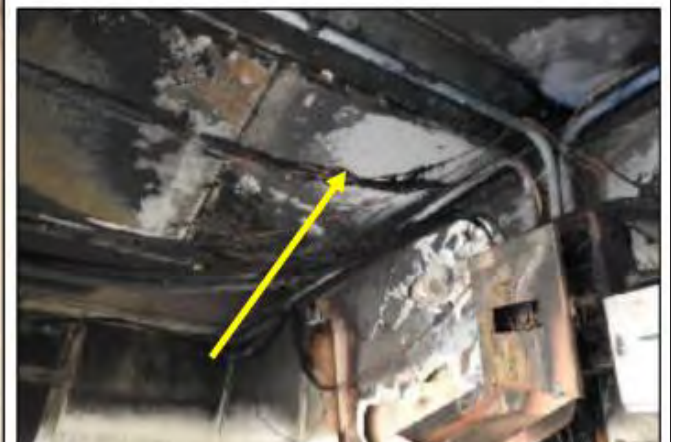
Ceiling panels to be examined for ACM's.
