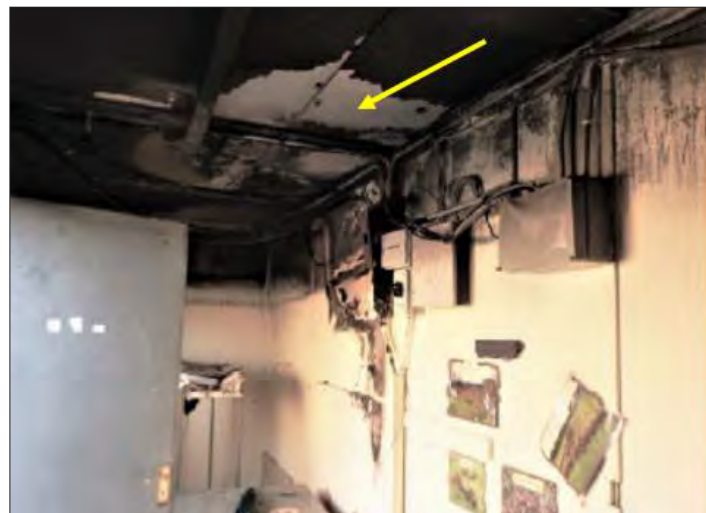
Entrance hall to the unit, now gutted from Electrical Fire damage.
