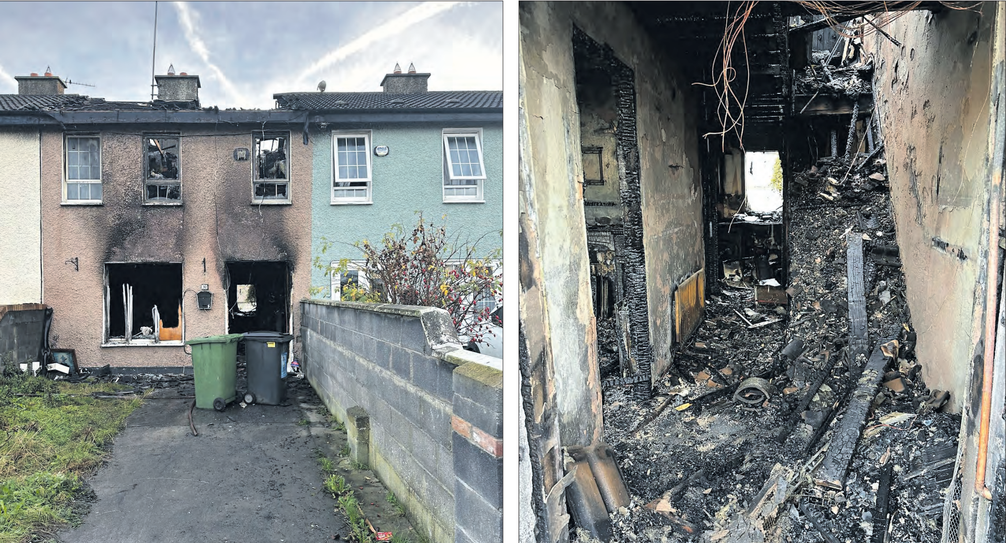
FIRE DAMAGE: The house in Quarryvale which was the target of a firebomb and (right) the inside of the property gutted
