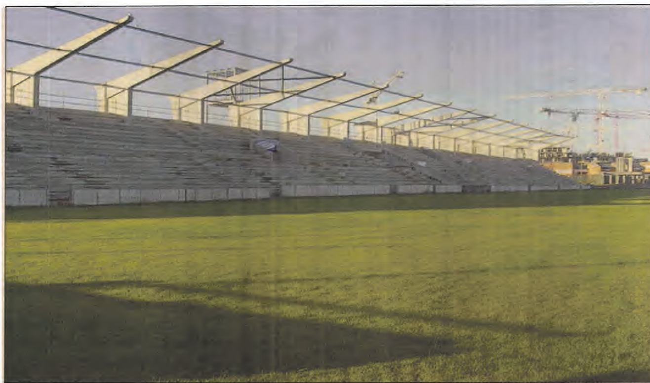
The half-finished Rovers stadium on the Tallaght bypass.
